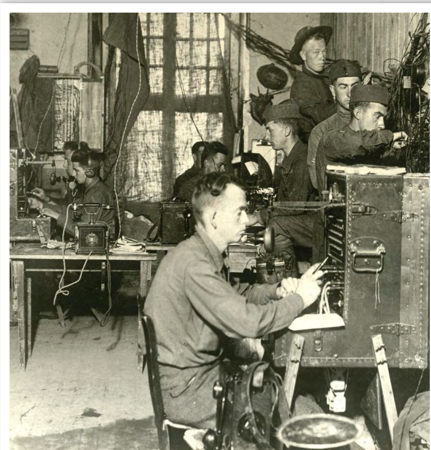
The American Field Signal Battalion's telephone switchboard in operation during the battle of St. Mihiel. Taken for Signal Corps USA, 1918. PCHS Collection, 2015.048.01221
